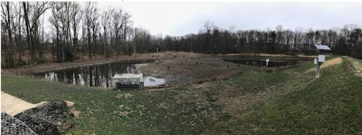
Stormwater Ponds days after rainy weather. The stormwater is retained and discharged after the water quality has improved and the water quantity has been reduced through infiltration and evaporation.
